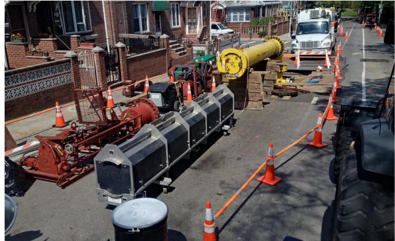
Brooklyn (NYC), NY - 20", 24", 30" pipeline inspection
